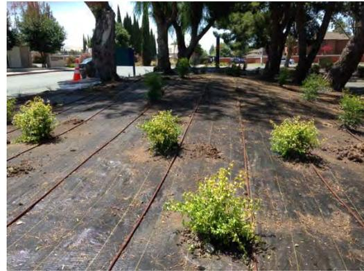
After turf was removed, the ground was covered with permeable weed barrier fabric to prevent weed growth, drip irrigation lines were laid on top of the weed fabric, and plants were installed through holes cut in the weed barrier. When planting was complete, the whole area was mulched with several inches of woodchips to conserve moisture and reduce weed growth on top of the weed barrier.
