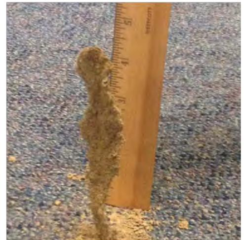
Subterranean termite tube emerging from a crack in the slab under the carpeting of a ground floor hallway at 597 Center in Martinez
